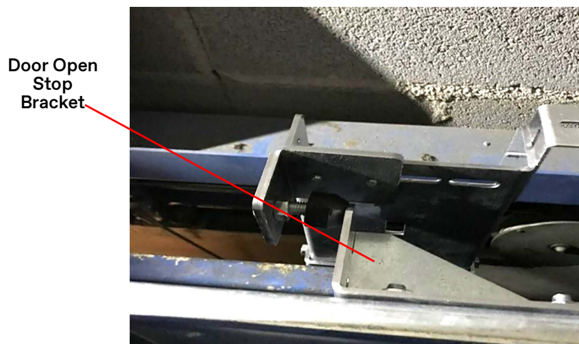
Figure 7- Door Open Stop Bracket Installation
