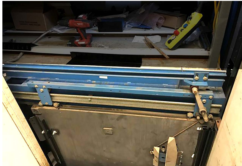
Figure 1 - Existing Door Operator Drive Components Removed Installation
