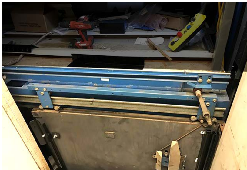
Figure 1 - Existing Door Operator Drive Components Removed
